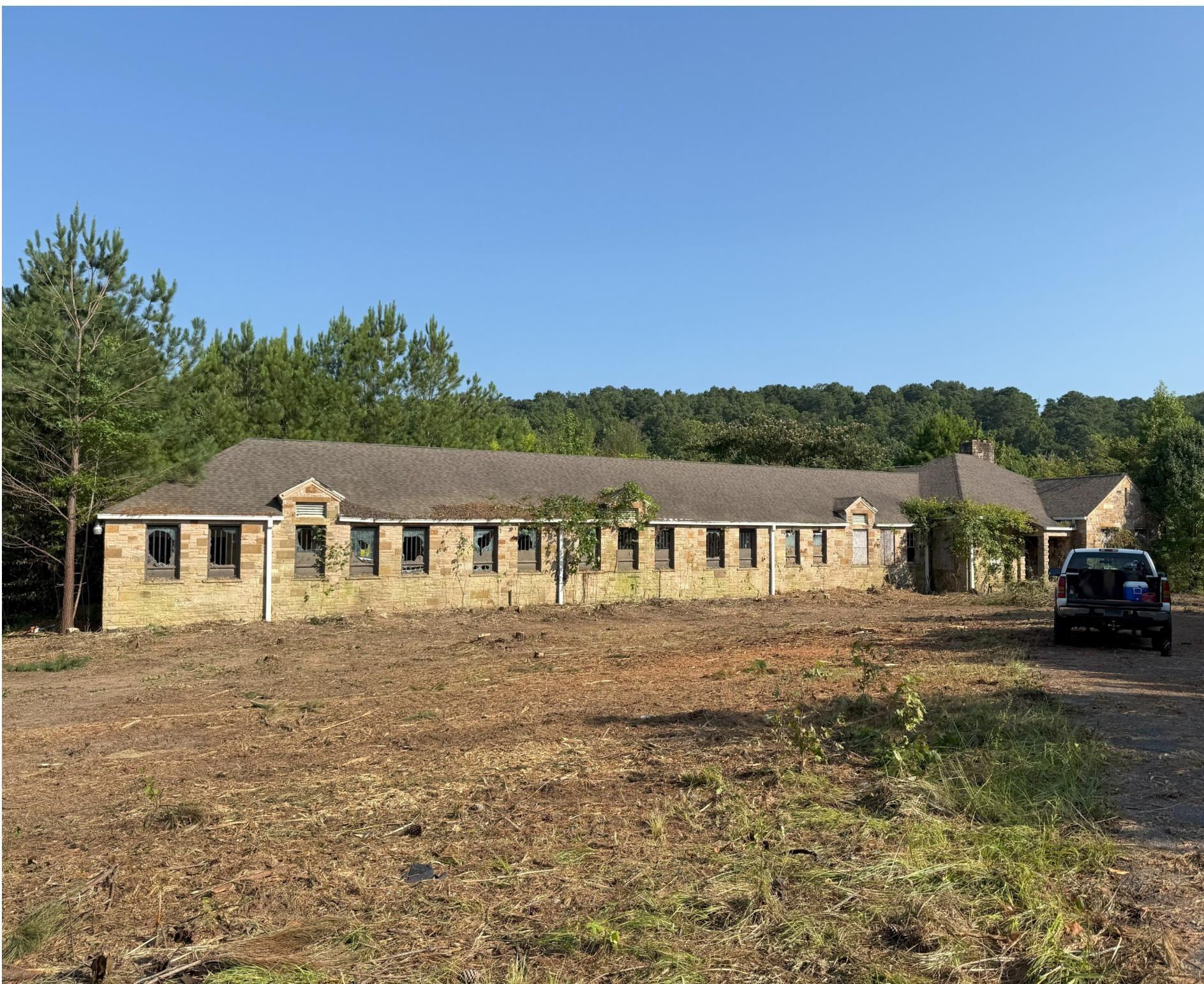
**This was a dormitory facility for the Alabama Girls' Reformatory. It was likely constructed in the 1930's. It is in fair structural condition and would need almost the entire roof structure replaced. Because of the layout of the building, it will be difficult to reuse.**
